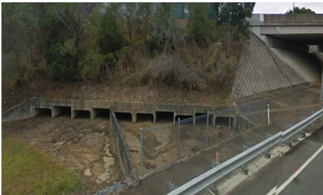
Culverts at Moreton Bay Road, facing downstream
