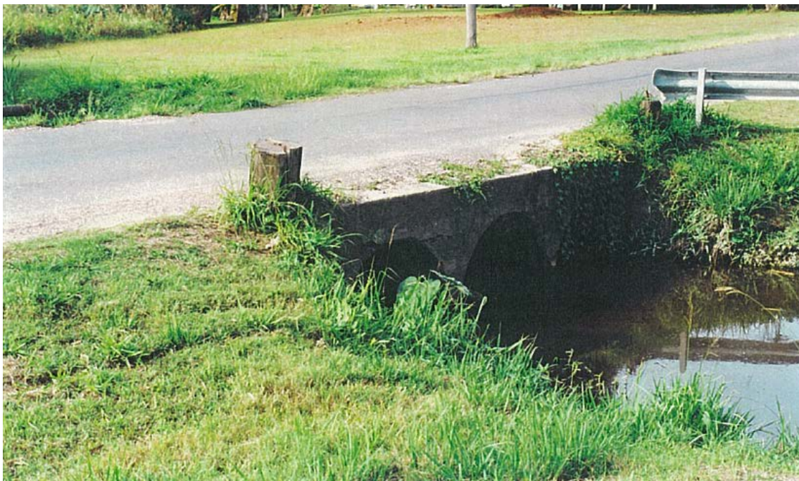
London Road crossing, facing downstream
