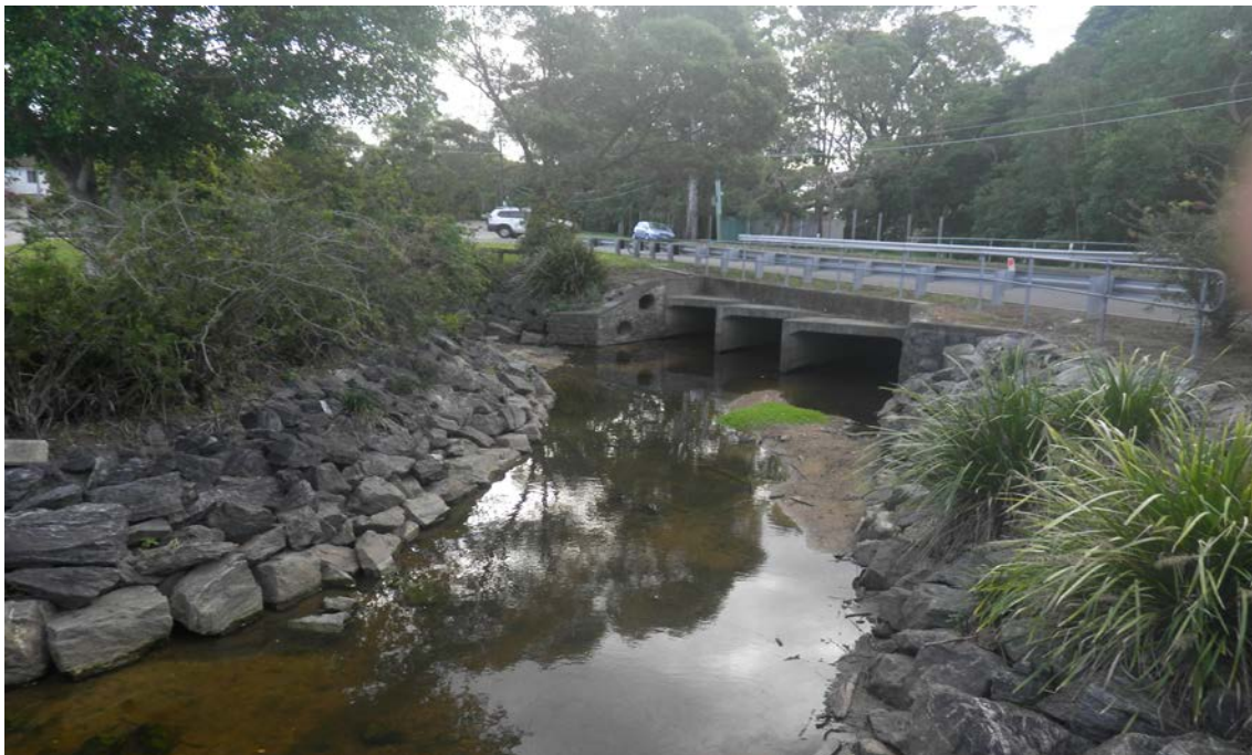
Culverts at Alexander Street, facing upstream
