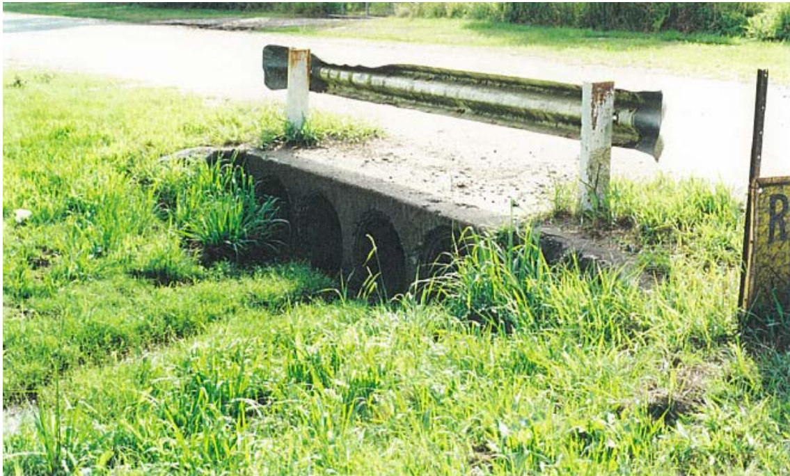
Boston Road crossing, looking downstream
