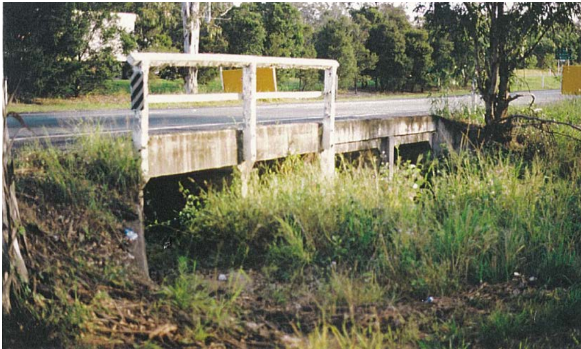
Old Cleveland Road Crossing, facing upstream
