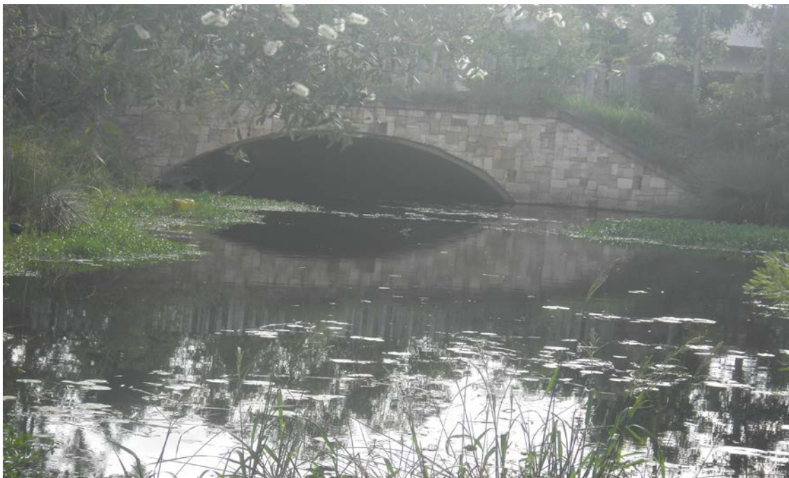
Bridge at Watervale Parade, facing downstream
