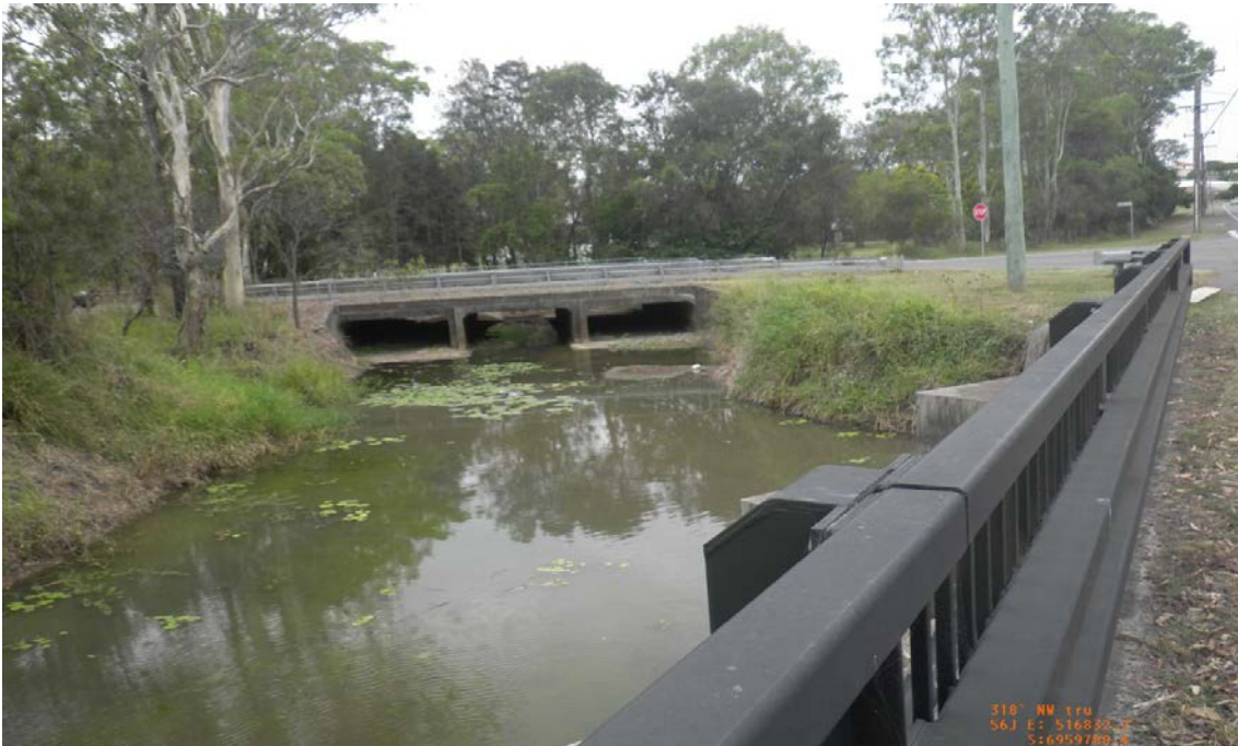
Culverts at Tilley Road, facing downstream
