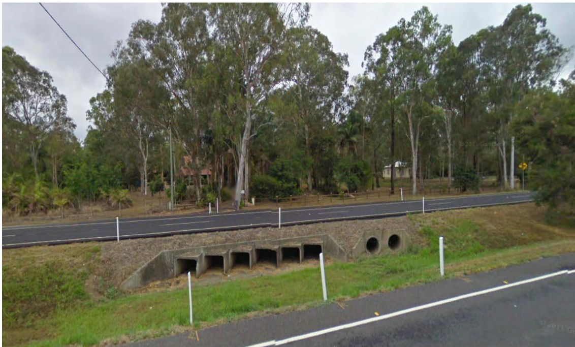
Culverts at Old Cleveland Road, facing upstream
