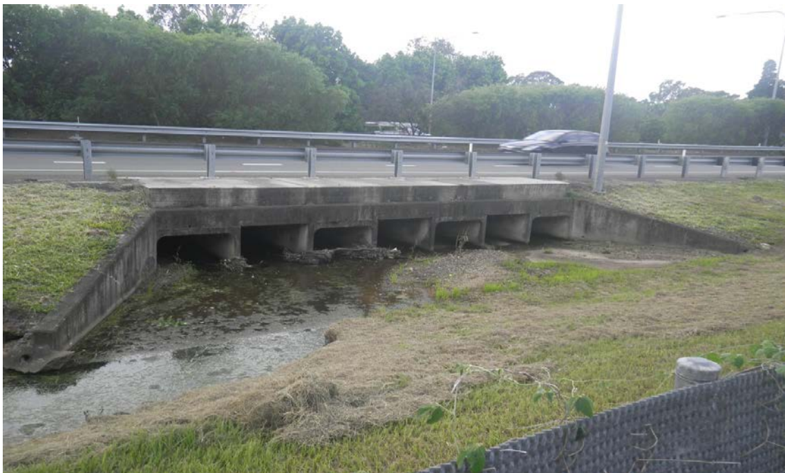
Culverts at Old Cleveland Road, facing upstream
