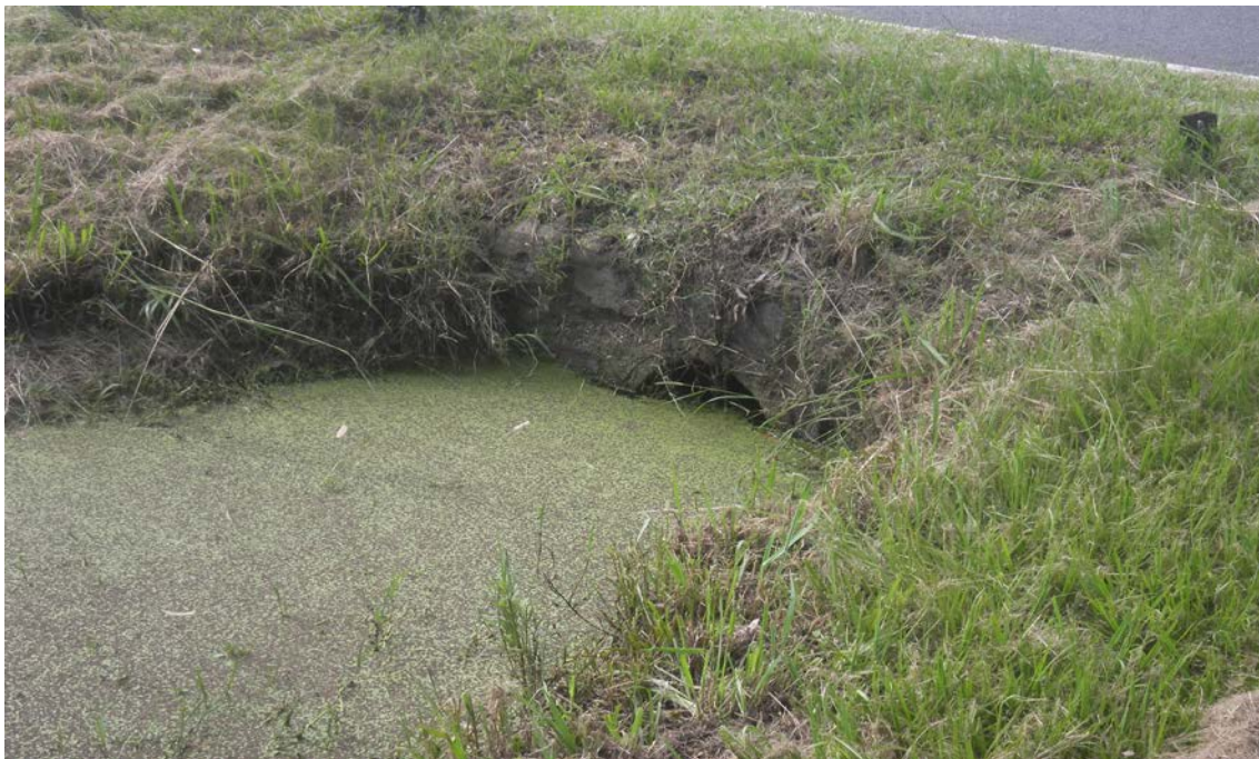
Culvert at Molle Road
