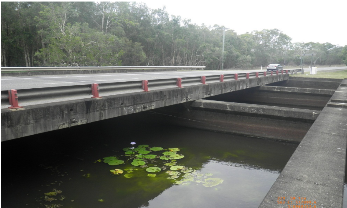
Culverts at Rickertt Road, facing downstream
