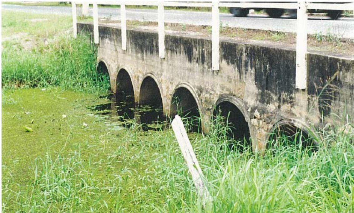
Culverts at New Cleveland Road, facing upstream
